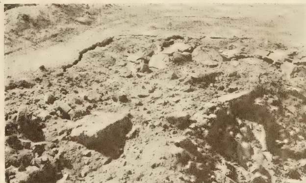
FIGURE 10.—FOR MOST SHALES, HARD-PANS AND PARTLY DISINTEGRATED ROCKS AN EXPLOSIVE HAVING A SLOW, HEAVING ACTION IS BEST. THIS 18-FOOT LIFT WAS THOROUGHLY BROKEN, ALTHOUGH THE ONLY SURFACE INDICATIONS WERE A FEW CRACKS AND A HEAVE OR BULGE ABOVE THE ORIGINAL GROUND LINE
